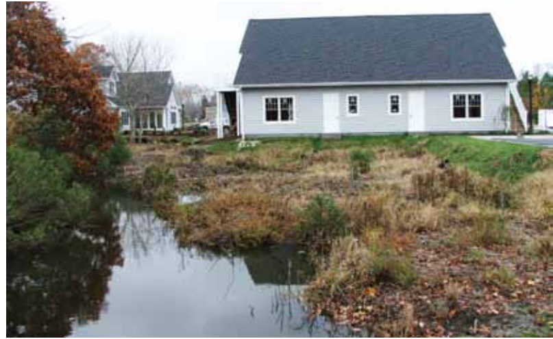
House built on very edge of tidal creek.
