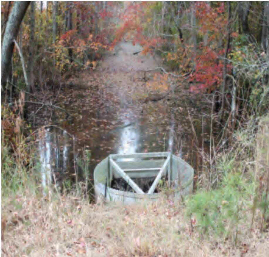
Once used to drain the swamp, rain-fed ditches have been plugged and fitted with gates (foreground) that can be raised to allow more water into the swamp.
