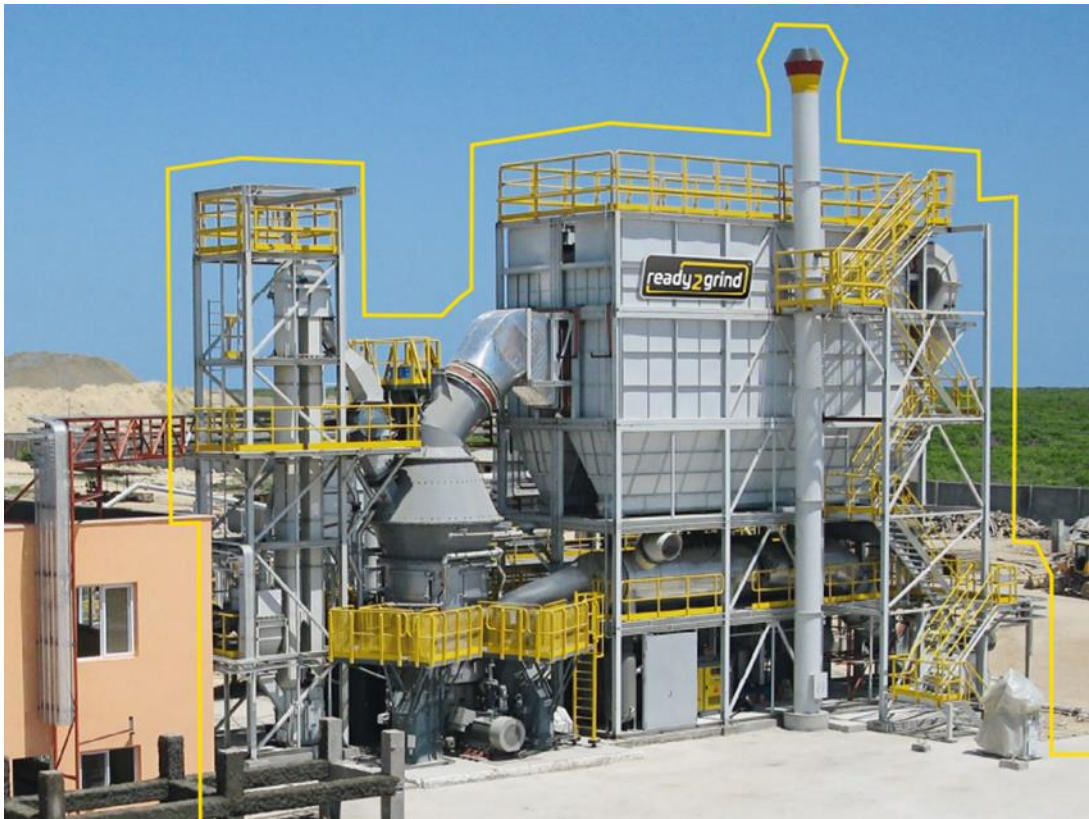
Grinding on the ready2grind system
