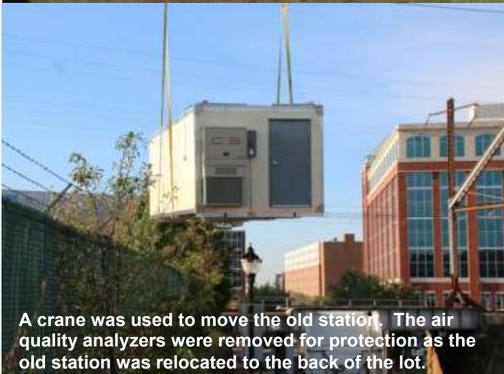
A crane was used to move the old station. The air quality analyzers were removed for protection as the old station was relocated to the back of the lot.
