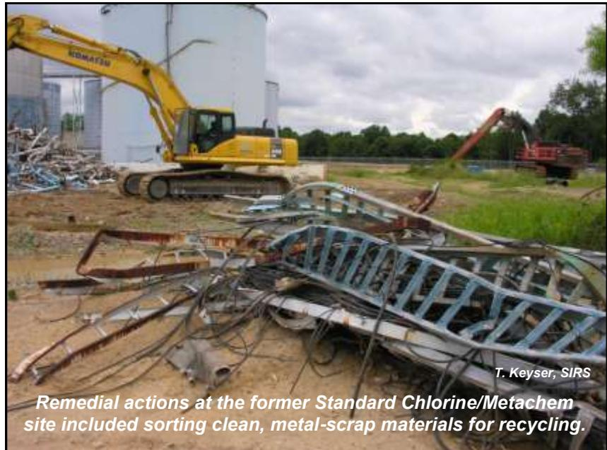
*Remedial actions at the former Standard Chlorine/Metachem site included sorting clean, metal-scrap materials for recycling.*
