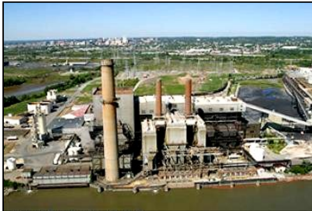
Connecticut Delmarva Generation-Edge Moor Power Plant —Conectiv, 2005
