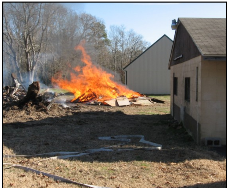
Open Burning of Construction Debris
