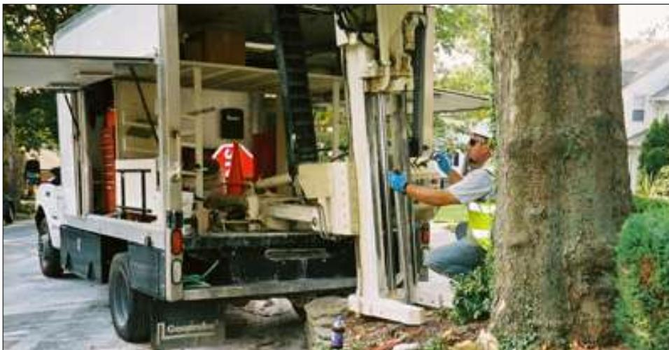
**A truck-mounted Geoprobe® was used for remediation injections in more accessible areas for the testing.**
