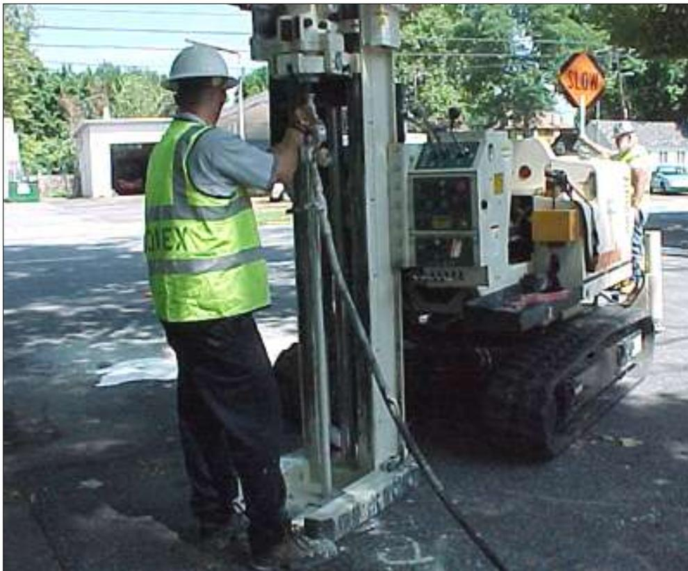
**A mini trackhoe-mounted Geoprobe® was used to inject an oxygen-releasing compound to remediate contaminated groundwater beneath Hillside Road.**
