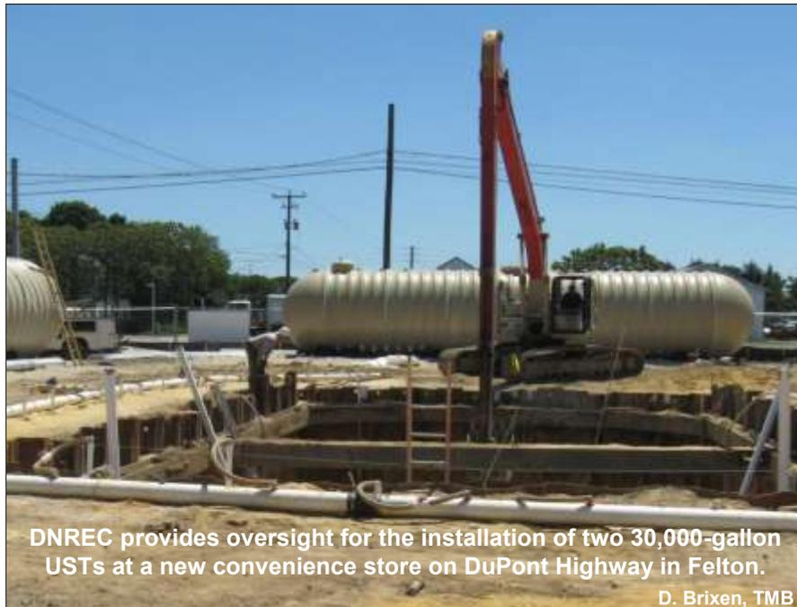
DNREC provides oversight for the installation of two 30,000-gallon USTs at a new convenience store on DuPont Highway in Felton.
