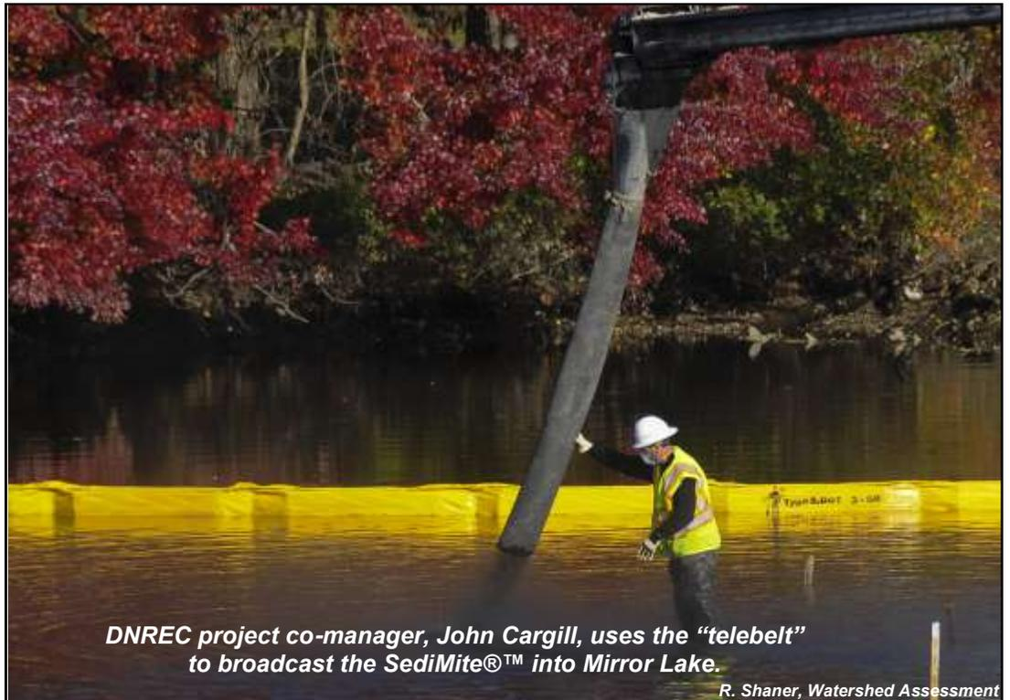
**DNREC project co-manager, John Cargill, uses the "telebelt" to broadcast the SediMite<sup>®</sup> into Mirror Lake.**
