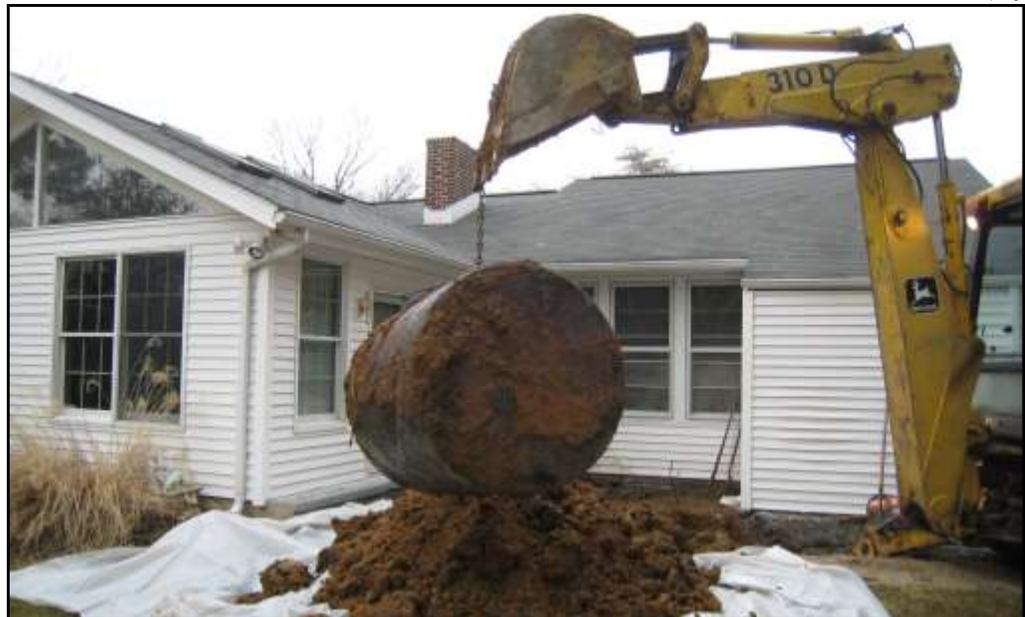
**A 300-gallon fuel oil UST is removed and staged on plastic at the Nicholson residence in Wilmington, prior to proper disposal by DNREC's subcontractor.**
