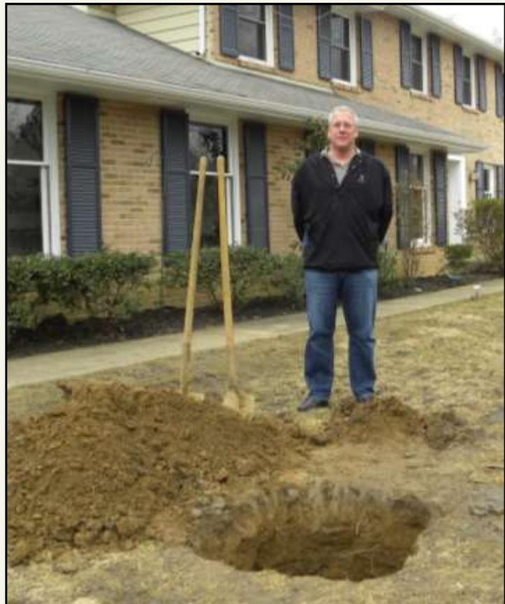
Newark homeowner, Steven Zabowski, observes the excavation of the abandoned 1,000 gallon UST located in his front yard. The top of the UST is exposed for cleaning and closure-in-place (by filling with concrete).
