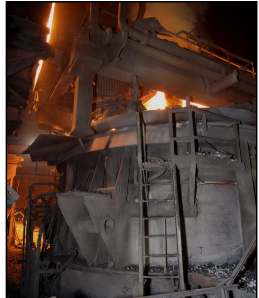
Claymont Steel's Electric Arc Furnace
