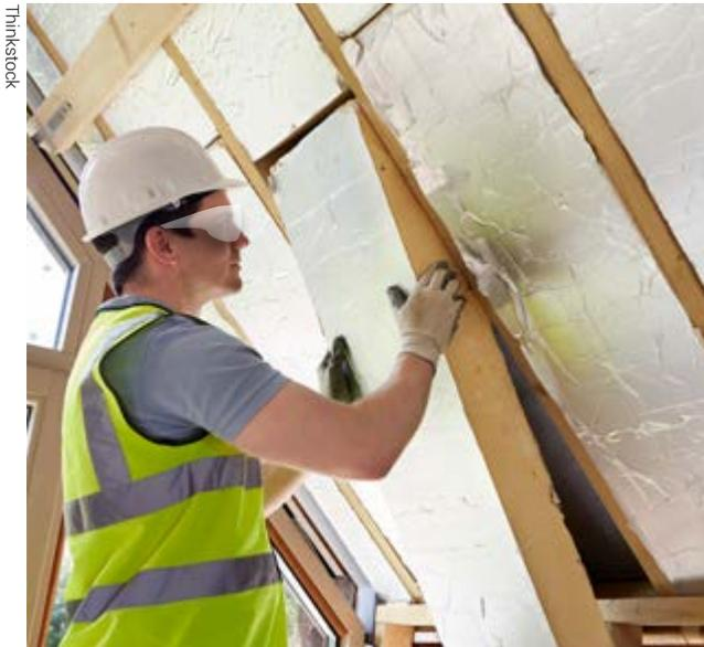
*A weatherization professional installs insulation panels into the roof of a home.*
