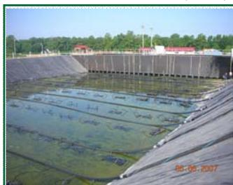
New Parkson Company Biolac® Wave-Oxidation® Biological Nutrient Reduction (BNR) Process equipment installed in existing Lagoon Number 3.
