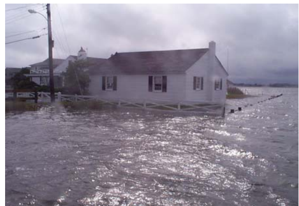
Flooding was minor and mostly of the nuisance variety.
