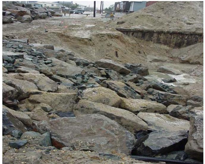
Stone Revetment to protect Ocean Drive and co-located utilities was constructed in early 2000.
