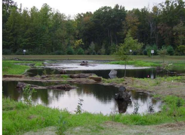
Field adjacent to existing stormwater basin and 46-acre wooded wetland was restored to a wetland. Water from the school's parking lots, building and fields is directed through the wetland before discharging into the stormwater basin.
