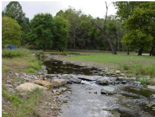
Before construction rip-rap was used in some areas to hold the stream banks in place (photo on left). The same area has been restored using logs, tree stumps, boulders, and live-branch willow layering to stabilize the banks and create habitat for fish and macro-invertebrate species.
