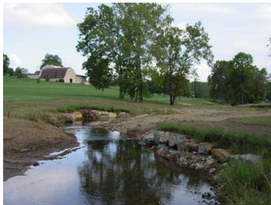
Stream banks have been stabilized and the sharp bends in the stream channel have been removed (photo on right). The pre-construction photo (left) shows a highly-eroded area with no main channel and banks that have been severely eroded and undercut.
