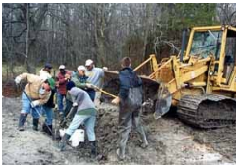
Students assist with installation of outlet pipe.
